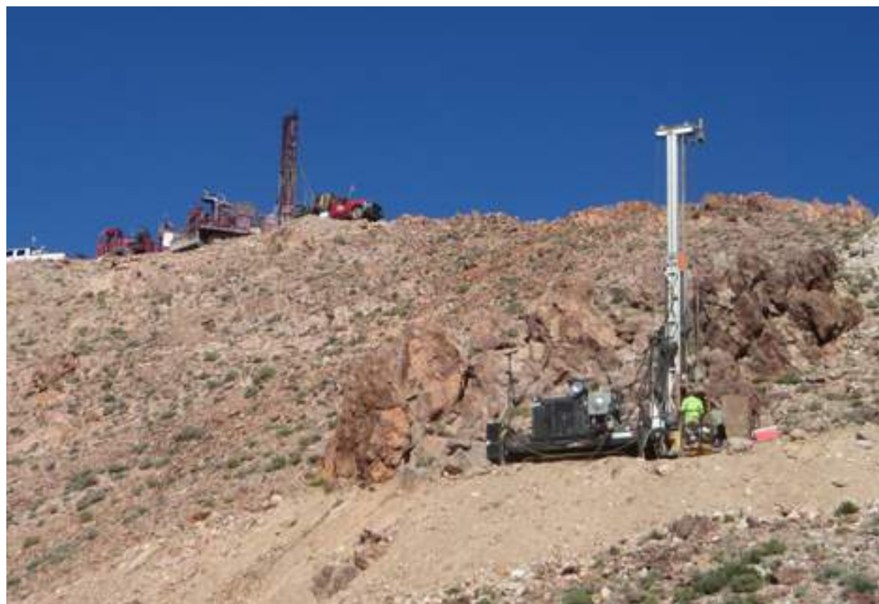
Photo: Drilling rigs at the Eastside gold project - Nevada
