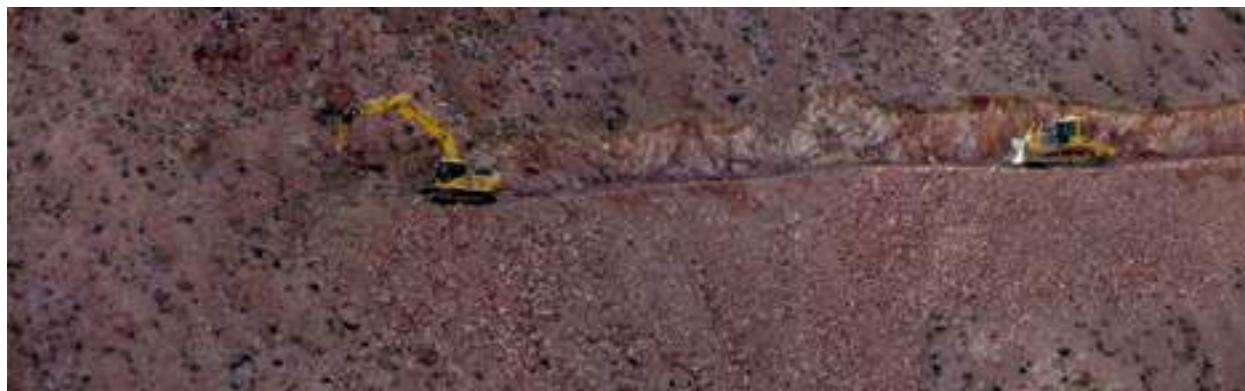
Photo: Road building - Eastside gold project - Nevada
